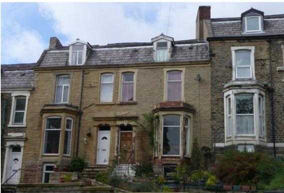
Figure 2 Original Windows replaced with inappropriate styles.
